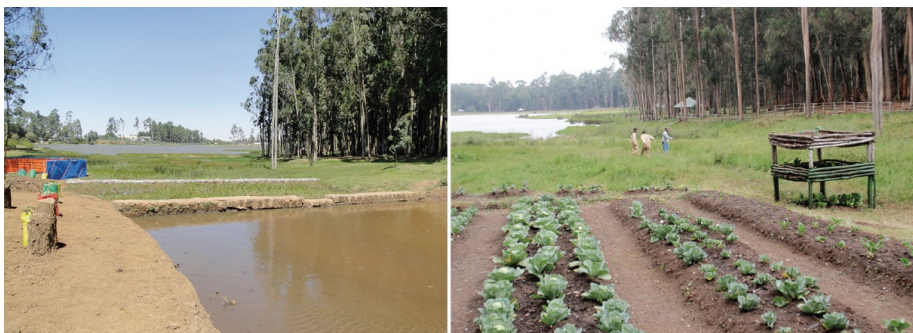
Figure 4. A sequential sedimentation-biofiltration system (SSBS) above the Burkitu reservoir in Assela Valley, Ethiopia (left) and the usage of sediments from SSBS as fertilizer
